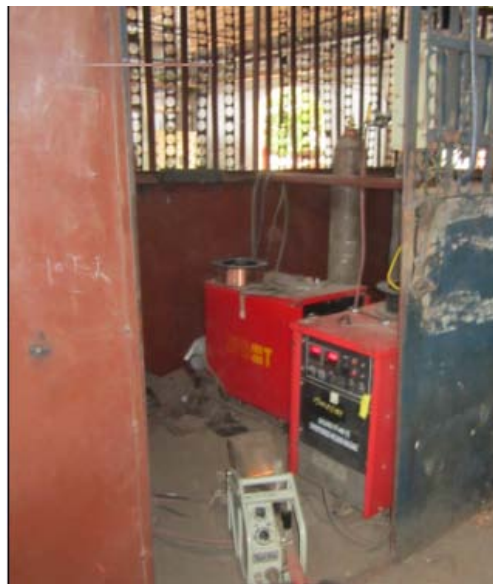
Figure 1: MIG welding machine setup
