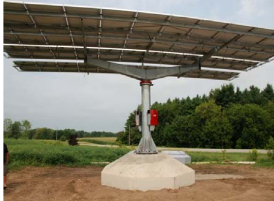
Figure 6: Double axis tracking system.
