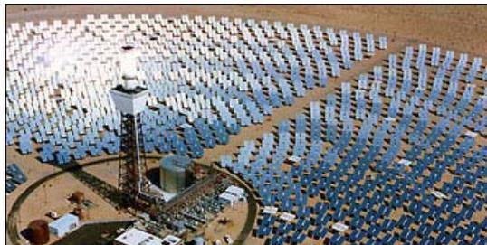
Mojave Desert. Component 2 is the central receiving tower, which receives the reflected radiation from the heliostats around it. The tower is installed with a boiler inside it. Component 3 is the power station, which is coupled to the solar collecting apparatus. The operation of the plant is as follows.
