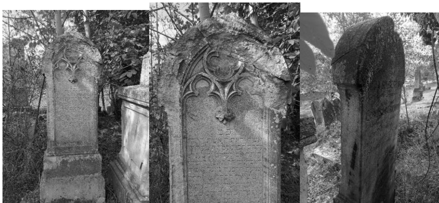
Fig.4: Gravestone with neogothic ornaments exhibiting cracking, scaling, delamination, biodeterioration
