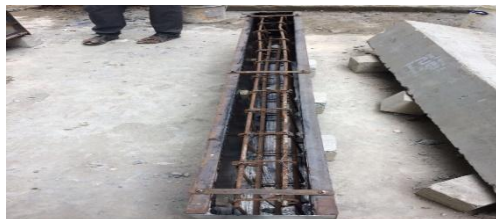
Fig. 4(a): Providing of Steel reinforcement in beam mould
