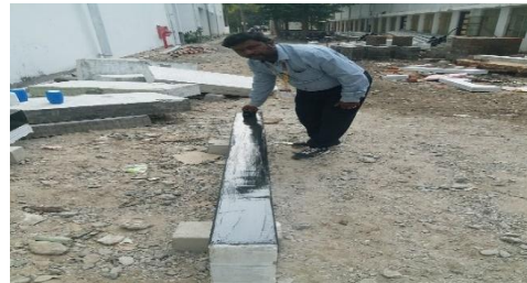
Fig. 4(c): Application of CFRP sheet
